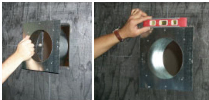
Wall Thimble - level & secure with 4 screws.
