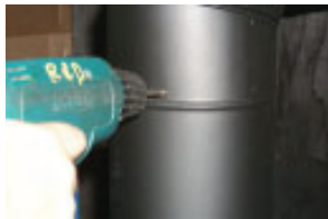
Secure 90° elbow to vertical pipe with Mill-pac and 3 screws.
