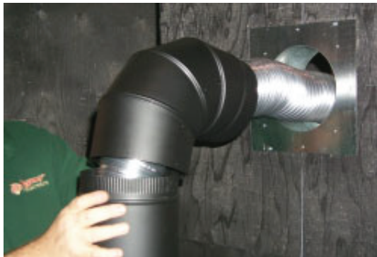
Slide 90° elbow over flex
